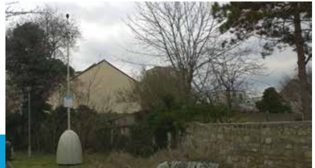
Station de Villeneuve-la-Garenne
